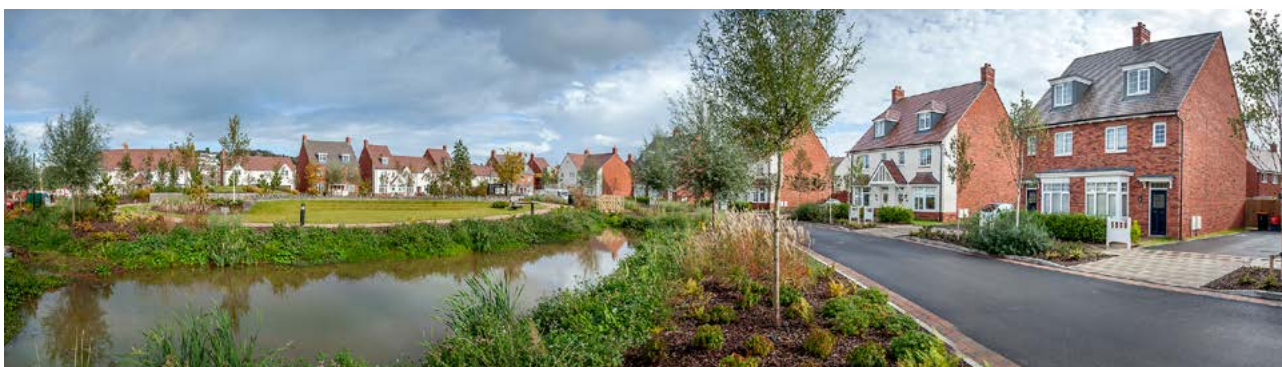
Housing overlooking landscaped park
