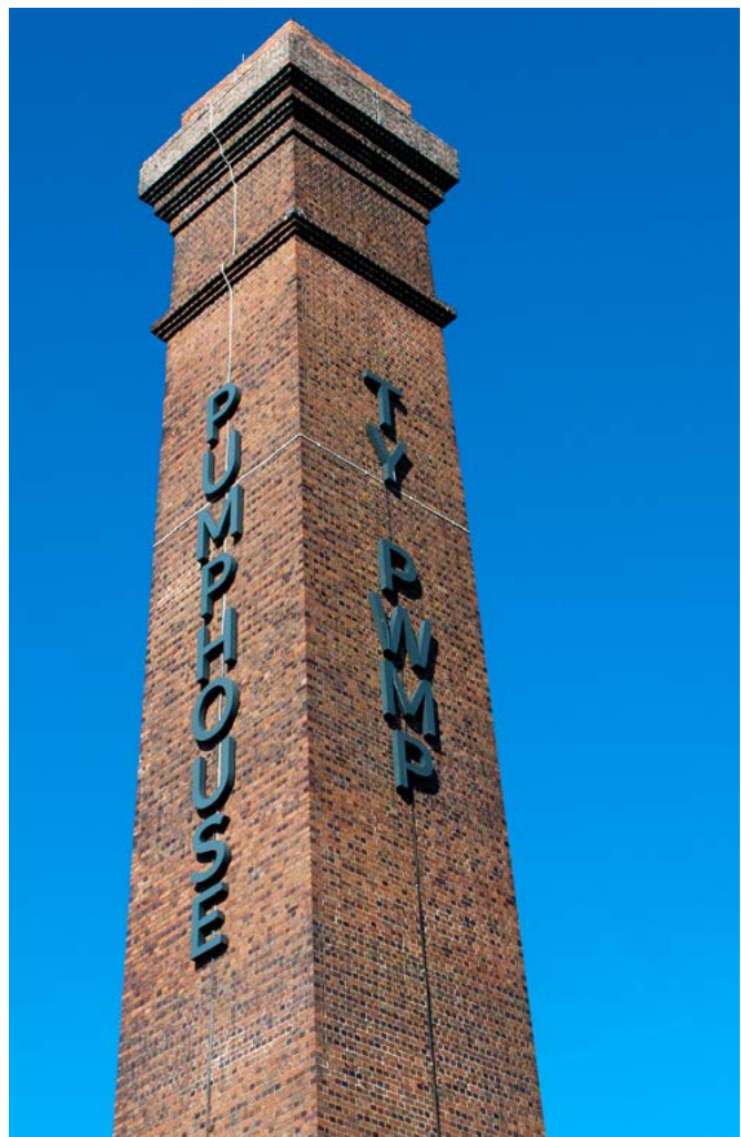
The Pumphouse Tower
