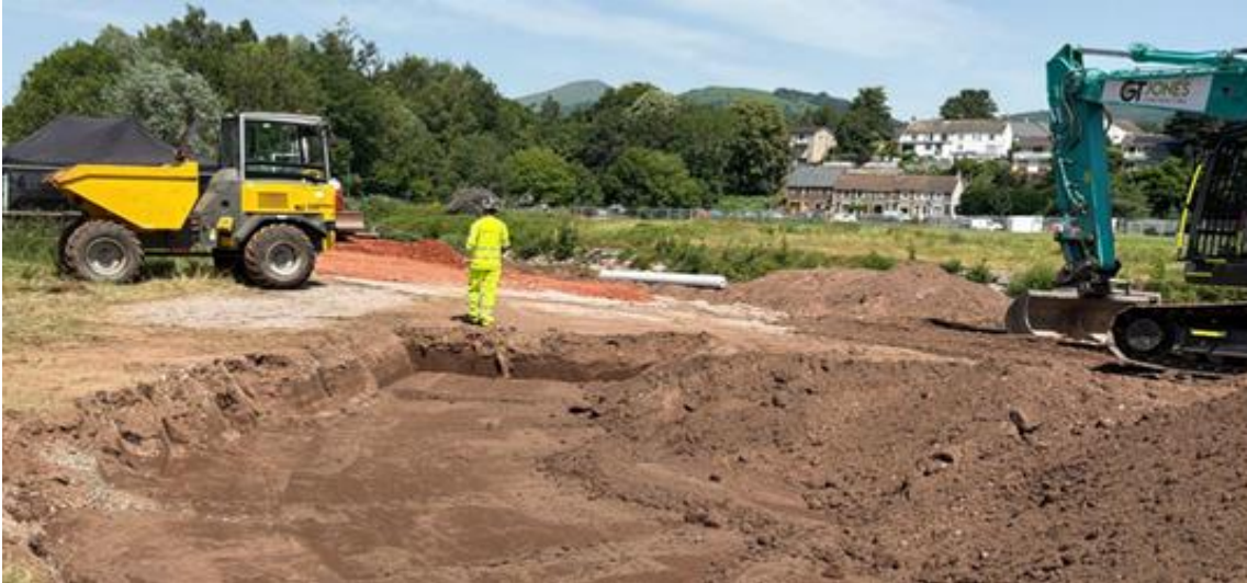
Stripping topsoil for the north access and piling platform
