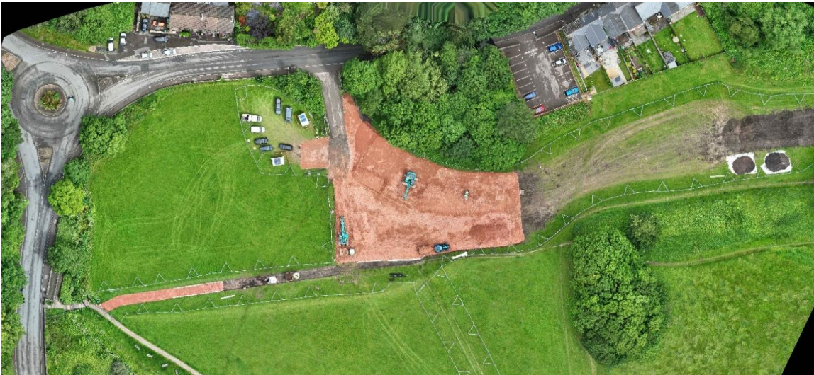
Balfour Beatty site compound preparation – Topsoil will be re-laid and reseeded at project completion
