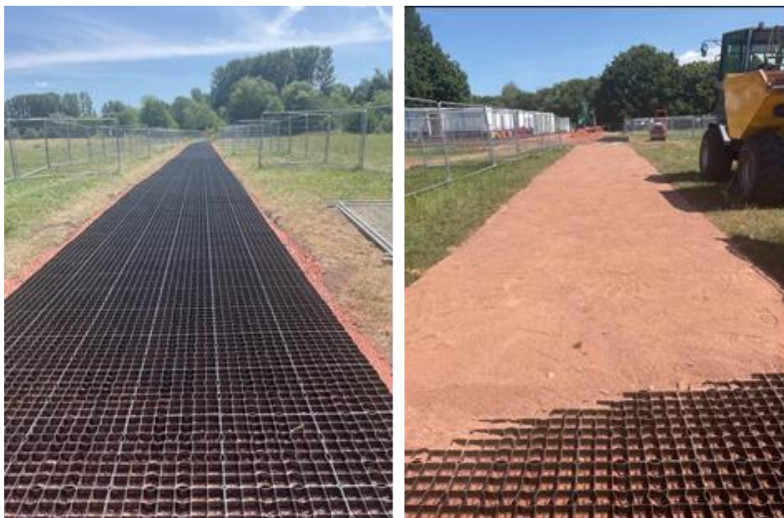
Preparing the PROW diversion
